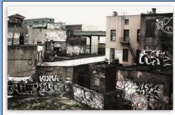
Spreading to other buildings (Urban Decay) ...
