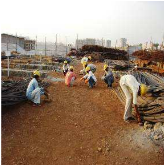
Safety violators putting in their effort to clear the steel rings
