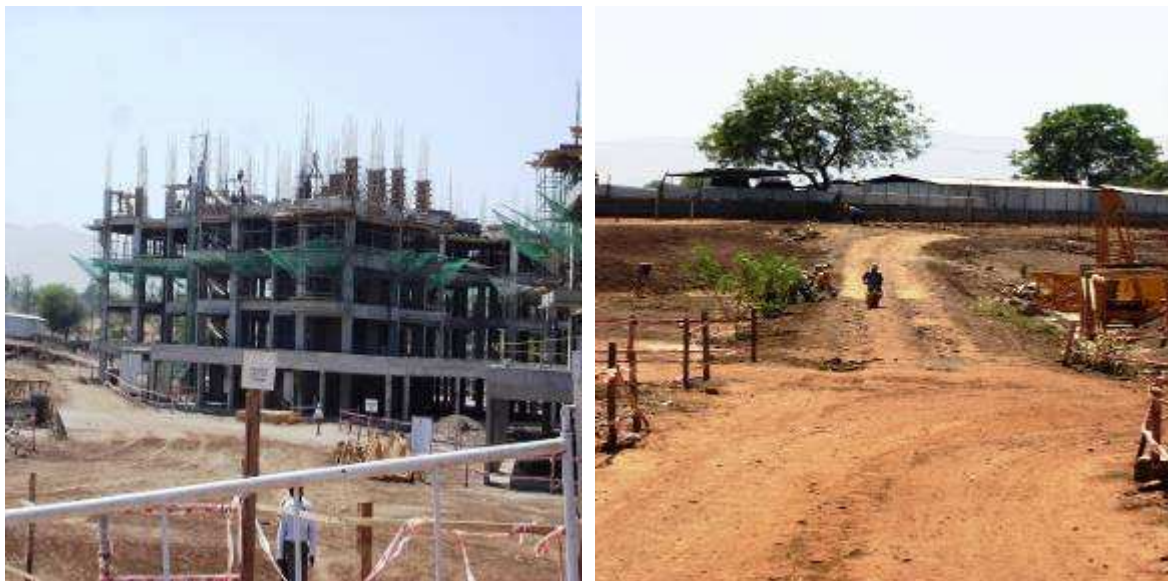
Labourers at the site before declare of emergency
