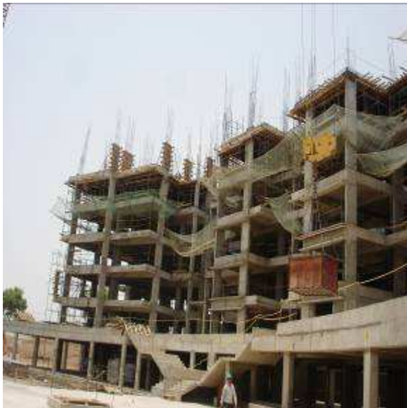
Work in progress before declaring Emergency
