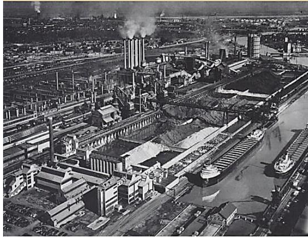
In about 1928, showing iron ore carriers in the northern end of the slip at the right and storage bins at the left of the slip. Further left are the blast furnaces, foundry, and power plant. Figure 2.5 The Rouge plant, world’s largest single-company industrial concentration (Lewis, 1987, p172)
