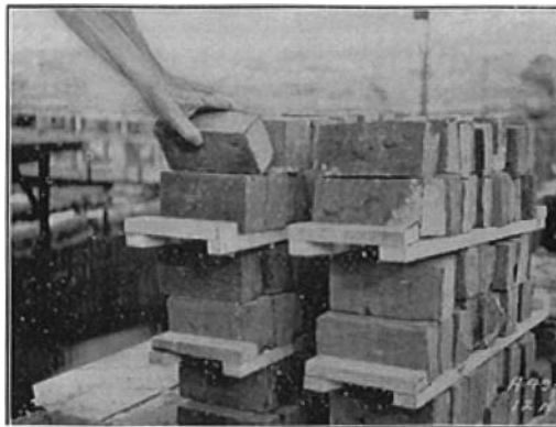
FIGURE 5.21 Gilbreth Bricklayers - Wrong Way to Pick Up a Brick. Source: Motion Study, Gilbreth, Hive Publishing © 1911.
