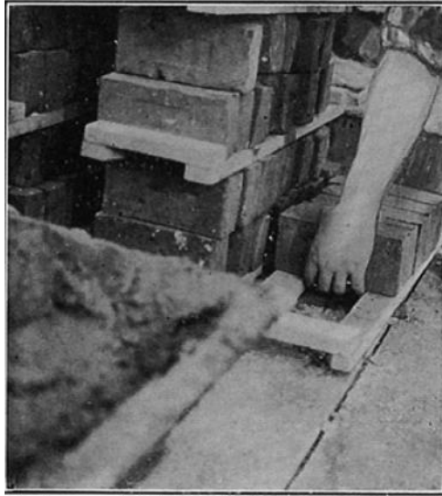
FIGURE 5.22 Gilbreth Bricklayers - Right Way to Pick Up a Brick. Source: Motion Study, Gilbreth, Hive Publishing © 1911.
