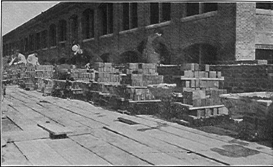
FIGURE 5.24 Gilbreth Bricklayers - Material Presentation After Material Handlers (or referred to as water spiders) made sure cement was always mixed properly so brick layers did not have to stop and could concentrate on just laying brick. He could construct buildings much faster than his competition so he won most of the bids. Source: Motion Study, Gilbreth, Hive Publishing © 1911.
